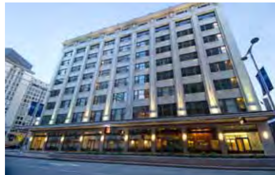
The Residences at 668 Euclid Project
